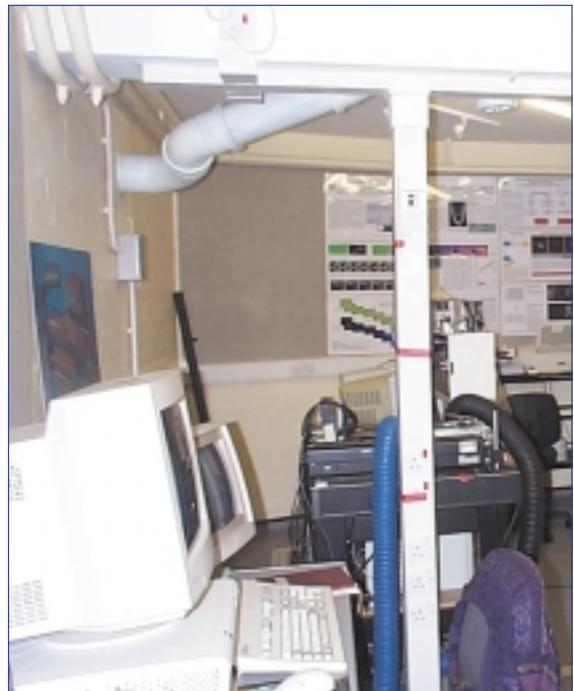
Each microscope should be installed on a sturdy table with free access all around ( $\geq 0.5\text{m}$ ) (see Fig 1). Trailing cables are minimised by post-mounted services (Fig 2), which should include:
